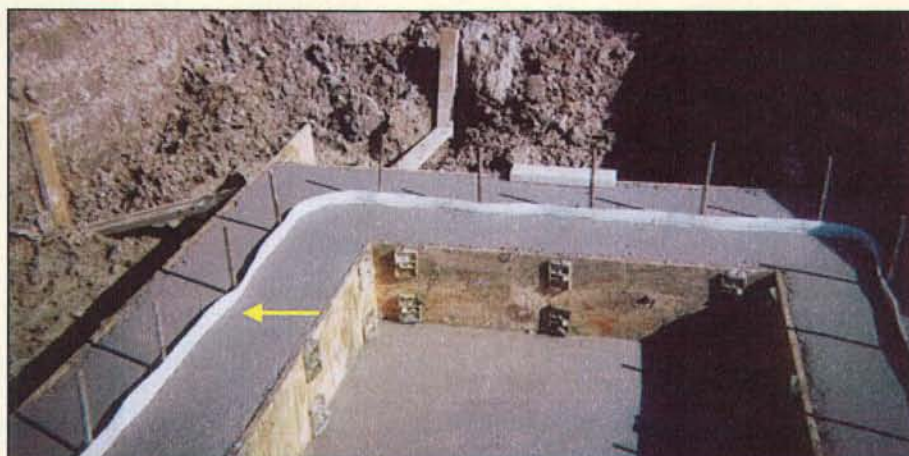
Water-proof barrier installed at all concrete joints to provide water tight seal
